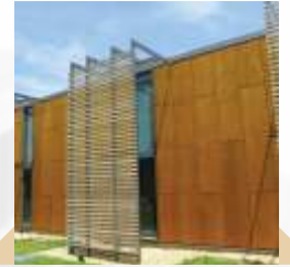
NATURAL WOOD FACADE
